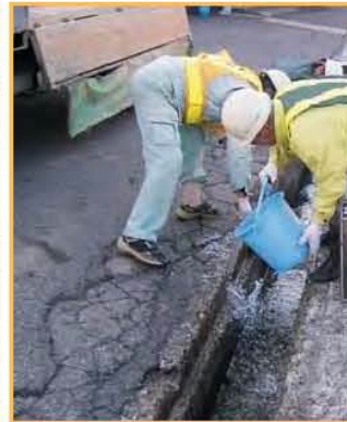
③ 既存側溝の清掃
