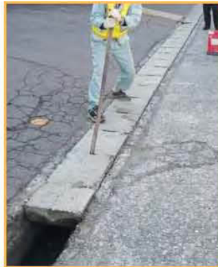
② 既存側溝の蓋撤去
