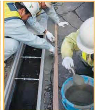
⑧ 既存側溝天端修繕
